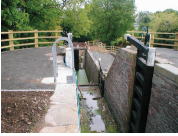
Locks 19-20 Prepared for a coat of paint
