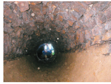
Culvert under towing path below lock 17
